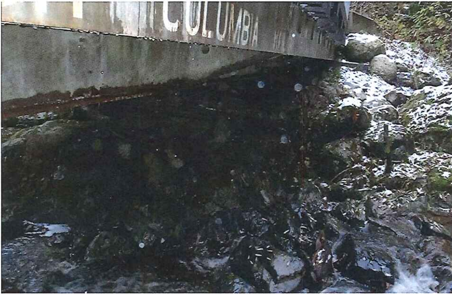
CK2441 Right Abutment
