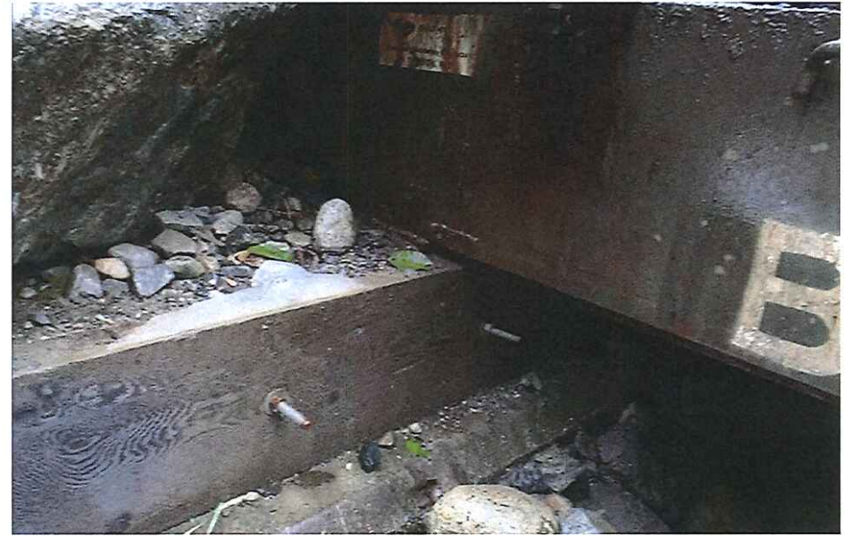
CK2441 Left Abutment Bearing
