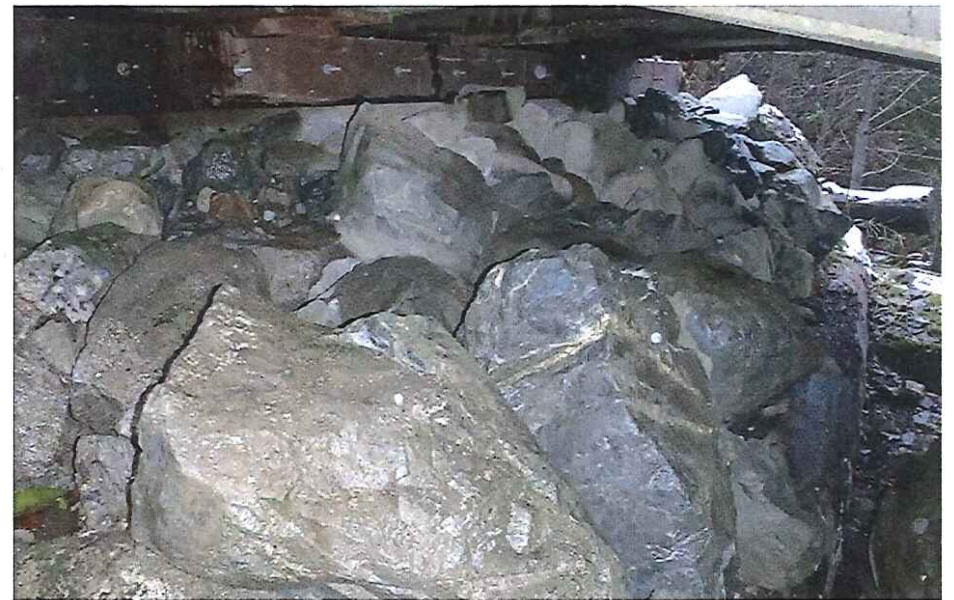
CK2441 Left Abutment
